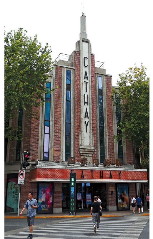
The Cathay Theater, a time-honored cinema on Huaihai Road, suspended operations for renovations this week. — Dong Jun
